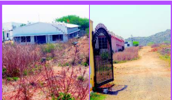
Malkapur Textile Park in a state of neglect
