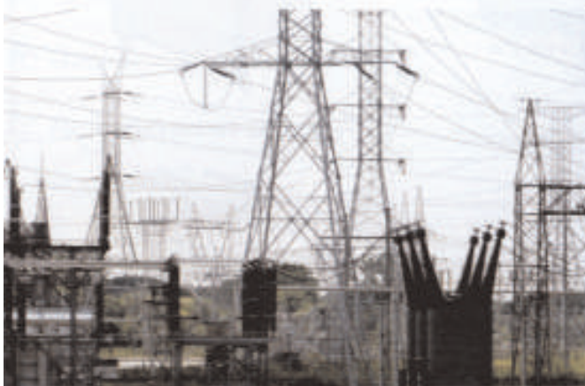
Transmission Line & Tower-erection projects
